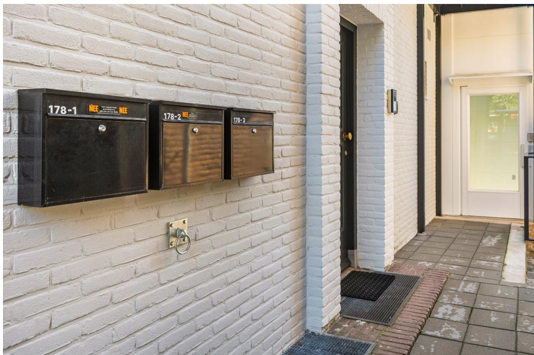
Entree begane grond
