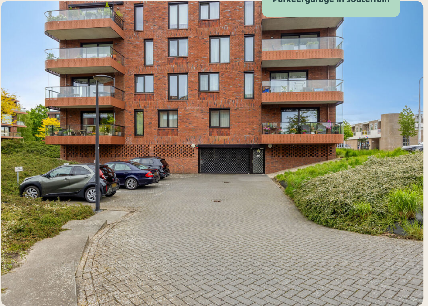
Parkeergarage in souterrain
