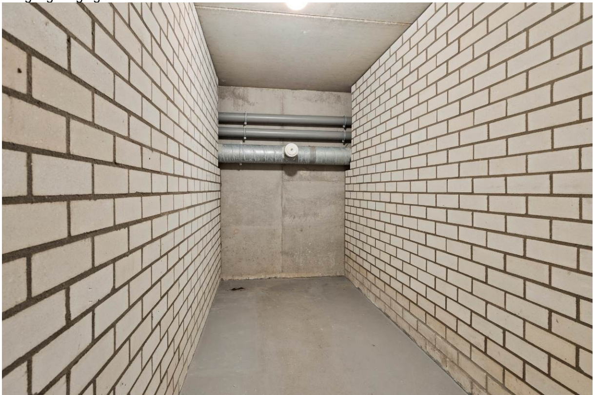
Berging in kelder
